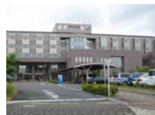
Figure 3 Kurihara City Central Hospital with SI, Miyagi prefecture
