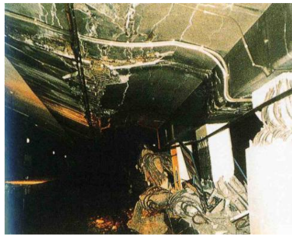
Photo 18 Collapsed center pillar and subsided upper floor slab of
