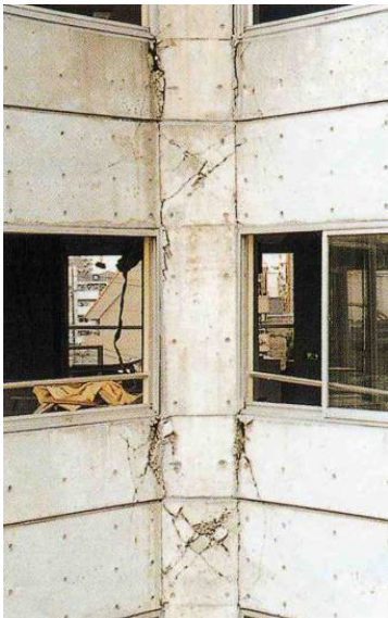
Photo 3 Shear cracking of exterior beam-column joint
