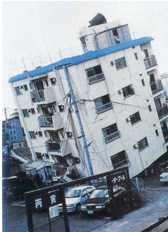
Photo 1 Building collapse at soft 1st story
