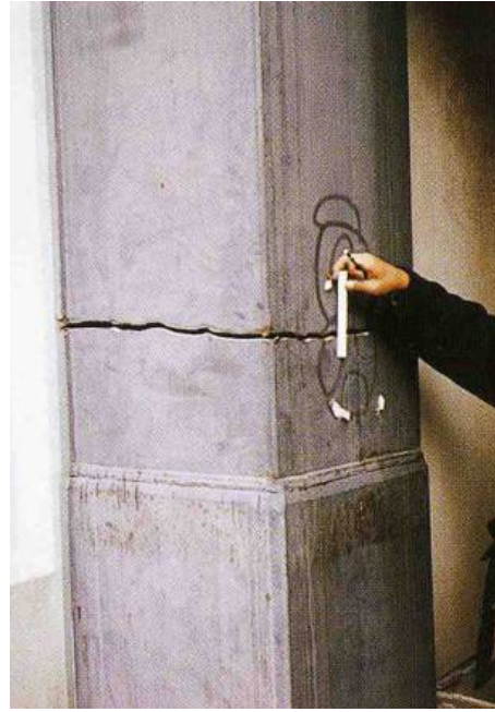
Photo 6 Brittle fracture of base metal in 1 st column of steel high-rise building
