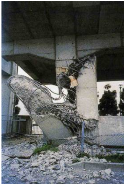
Photo 15 Shear failure of railway RC-frame
