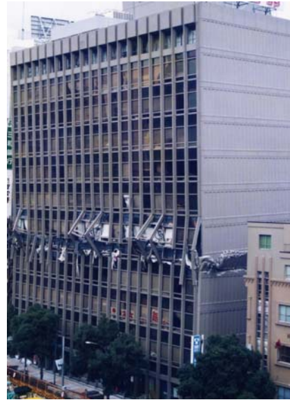
Photo 9 Story collapse at 5 th floor
