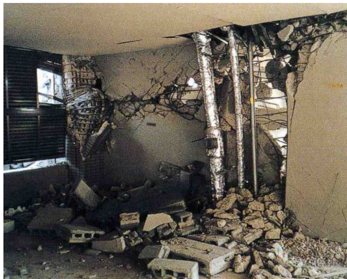
Photo 4 Sliding shear failure of wall at mid-height
