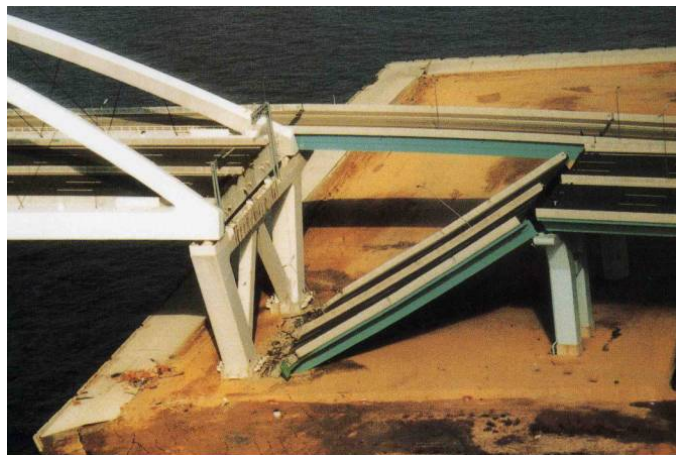
Photo 16 Fallen span in port bridge
