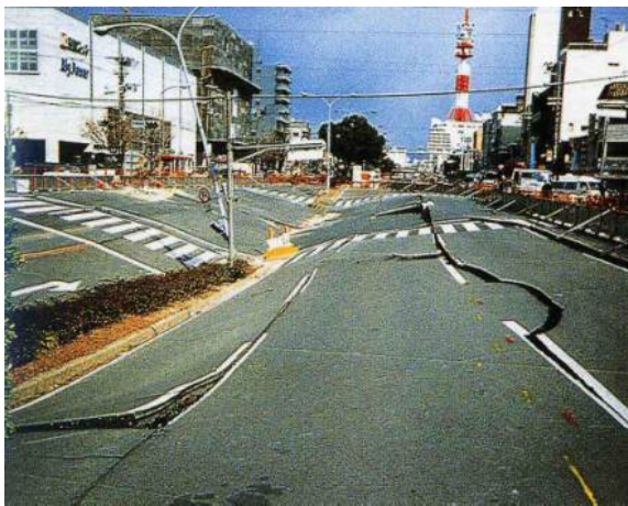
Photo 17 Settlement of national road over a subway station
