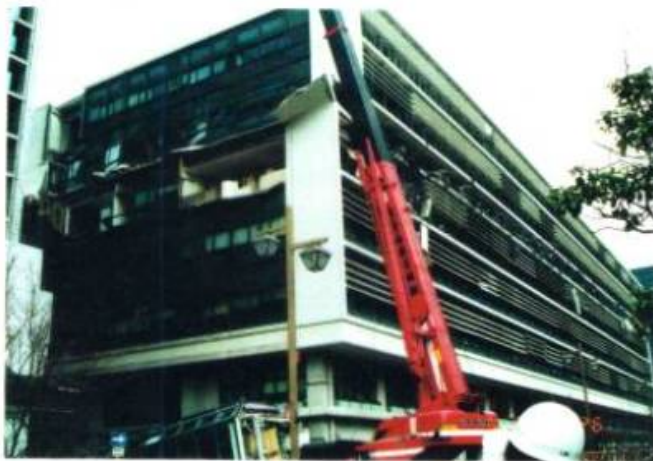
(a) Story collapse
