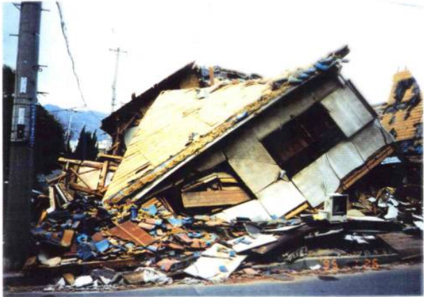
Photo 10 Collapse of old wooden house
