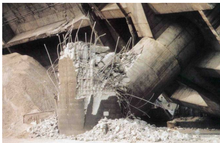
Photo 14 Shear failure of RC Pilz-type bridge
