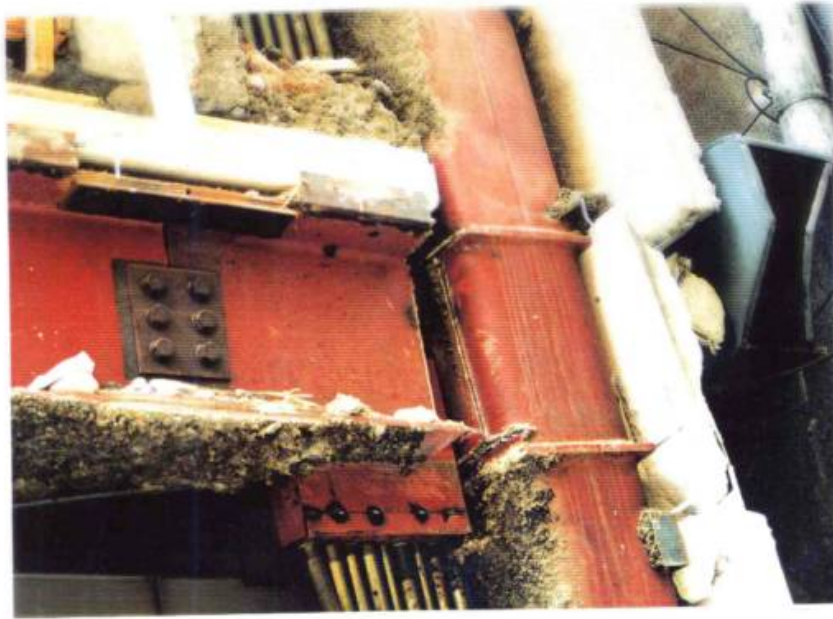
Photo 7 Damage to column-to-beam connection
