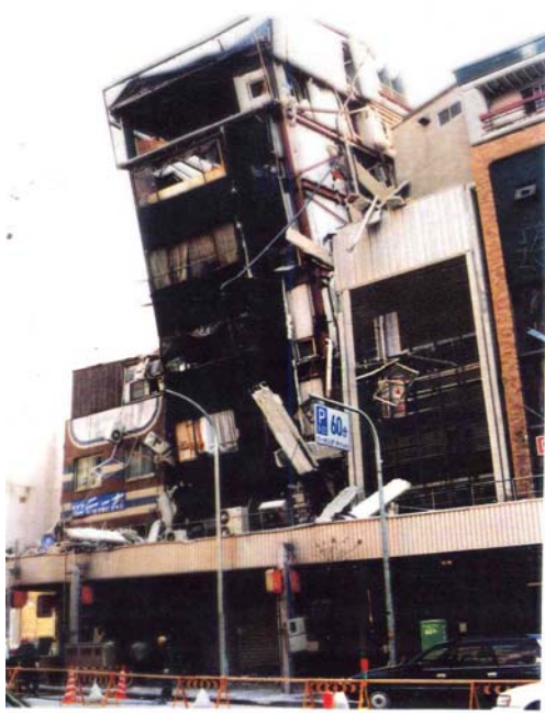
Photo 5 Steel-frame building with fracture of bracing members
