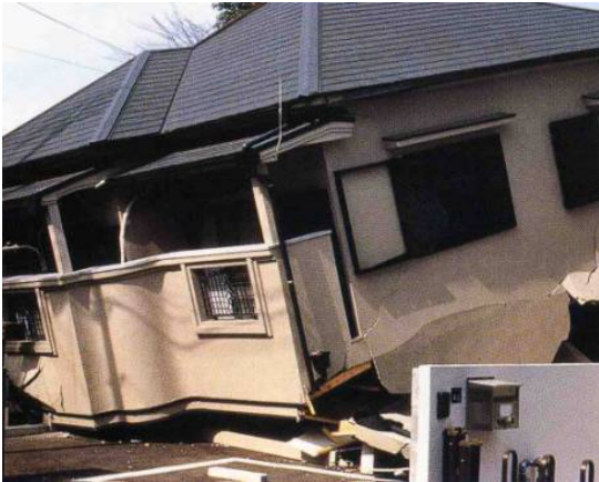
Photo 11 Collapse of new wooden house with garage
