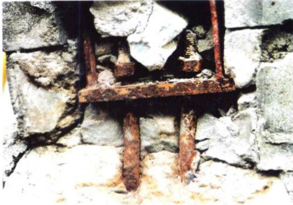
Photo 8 Pull-out of anchor bolts at column-to-base connection
