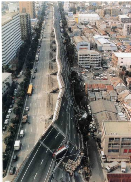
Photo 13 Damage to elevated urban highway (contributed by Yomiuri Shimbun)
