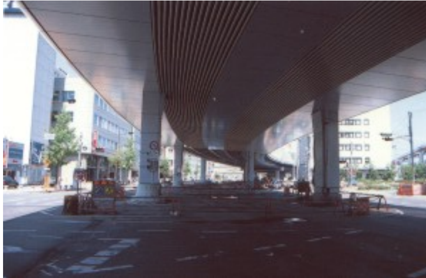
Photo 9 Benten viaduct after reconstruction
