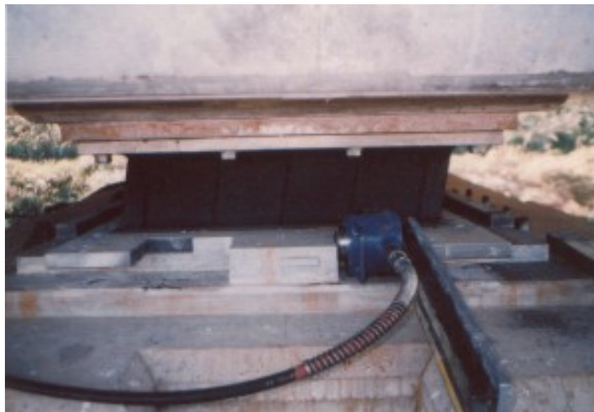
Photo 4 Repositioning of lower plate, Ohito viaduct
