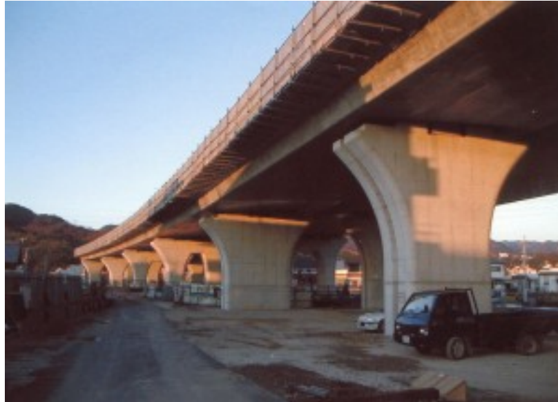
Photo 5 Wakayama bypass viaduct
