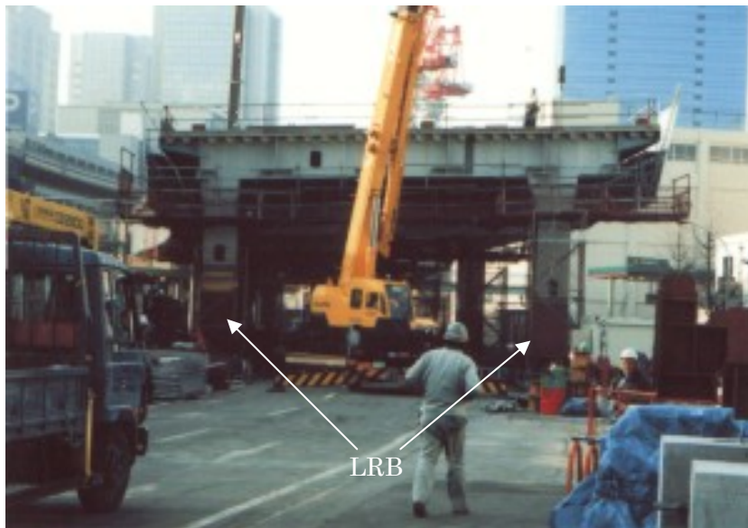
Photo 8 Lead rubber bearings installed under the bottoms of a steel frame
