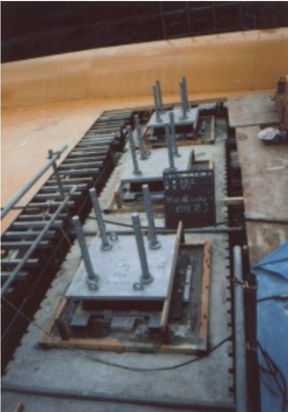
Photo 2 Lead rubber bearings, Ohito viaduct
