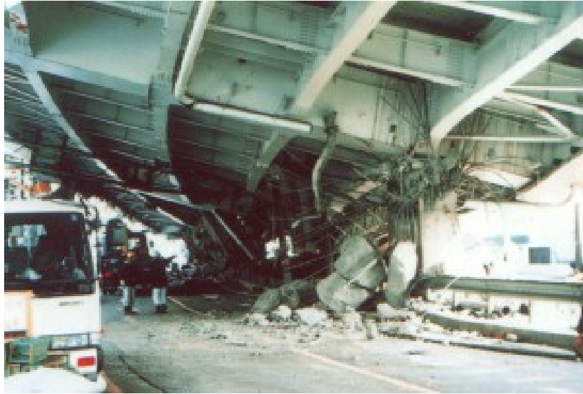
Photo 7 Collapse of Benten viaduct, Route 3, Hanshin Expressway, in the 1995 Kobe earthquake
