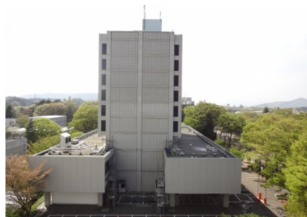
Photo 2 Damaged building viewed from the east side
