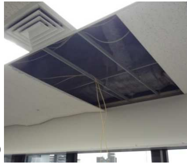
Fig. 3a Falling of the ceiling panel (28 th floor)
