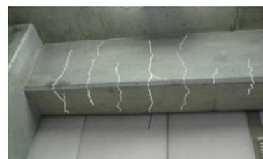
Photo 2.4. Cracks on girder.
