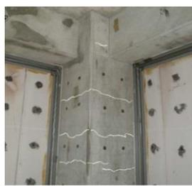
Photo 2.3. Cracks on column.
