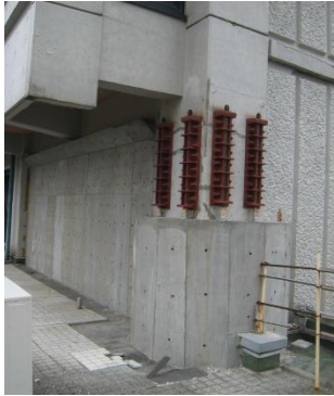
Photo 2.3 Emergency rehabilitation (on third floor)
