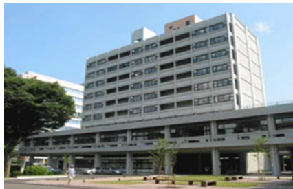
Photo.2.1 Building selected for study
