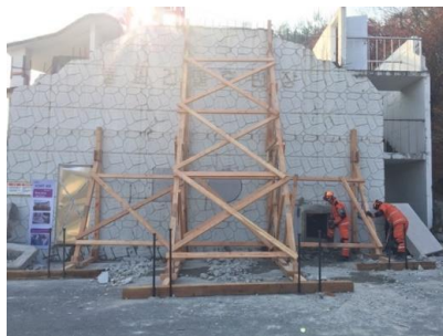
Photo 1 Example of Shoring 15
