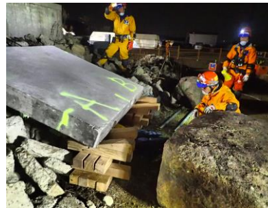
Photo 2 Example of Cribbing 16
