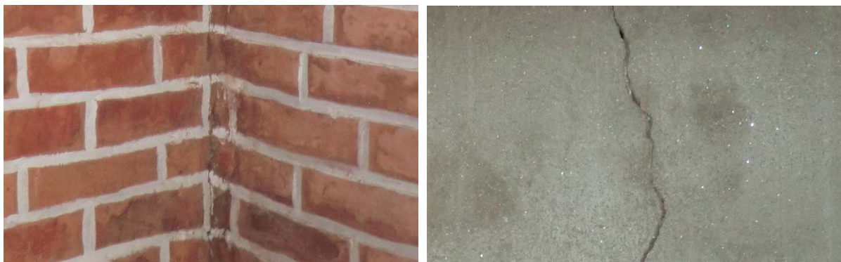
(a) Crack at D1
