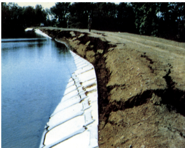
Photo 1 Cracks on the embankment and sliding of the sticking block [Reference 9)]
