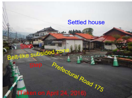
Photo 3 Damage in the Kario district
