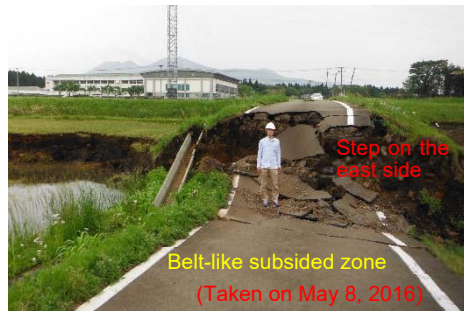
Photo 5 Damage in the Matoishi district
