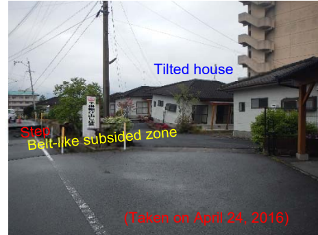
Photo 2 Damage in the Uchinomaki district
