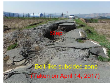
Photo 7 Damage in the Yakuimbaru
