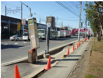
(Mihama 2, Urayasu, captured on March 18, 2011) (Takasu 7, Urayasu, captured on March 18, 2011) Photo 2 Sidewalk subsidence caused by liquefaction
