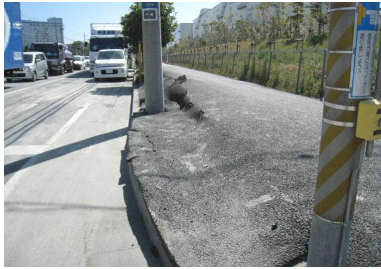
(Chidori, Urayasu, captured on March 18, 2011) (Maihama, Urayasu, captured on March 18, 2011) Photo 1 Raised sidewalk due to liquefaction
