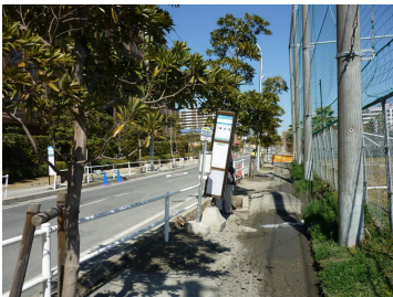
(Mihama 2, Urayasu, captured on March 18, 2011) (Takasu 7, Urayasu, captured on March 18, 2011) Photo 2 Sidewalk subsidence caused by liquefaction
