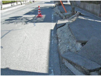
(Chidori, Urayasu, captured on March 18, 2011) (Maihama, Urayasu, captured on March 18, 2011) Photo 1 Raised sidewalk due to liquefaction
