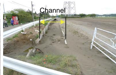
(c) 2011 sand boils filled up a channel (see Fig. 6(b) for location)
