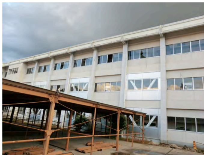
Photo. 1 North side view of the class-room building
