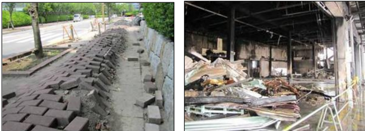
Fig. 7 Underground utility impacts due to soil liquefaction in Chiba (Tokyo metropolitan area) (left), and fire-following earthquake impacts at Sendai Airport cargo area (right) (Pierepiekarz)
