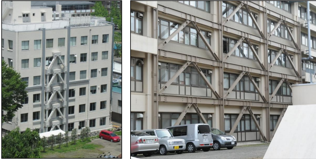
Fig. 4 Retrofitted buildings in central Sendai (left) and Tohoku University (right) (Siu)
