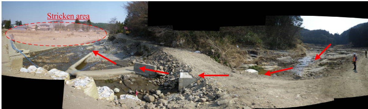
Photo 8 Path way of debris flow and downstream stricken area (April 15 th at 37.308131, 140.202481)
