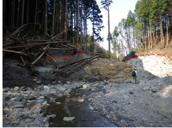
Photo 5 Mark of debris flows on valley walls (April 15 th at 37.306236, 140.199503)
