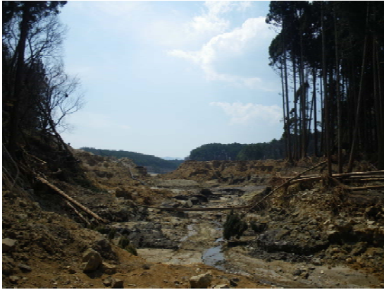
Photo 4 Breached dam body from downstream (April 15 th at 37.302661, 140.196055)
