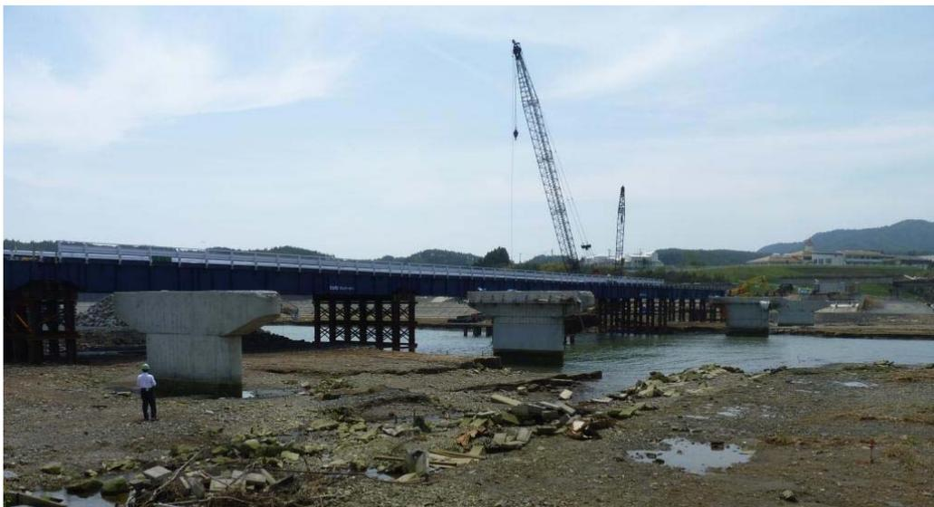
Fig.5 Remaining piers of Koizumi Bridge shown at low tide. Temporary bridge is under construction on seaward-side of bridge (photo: E. Monzon)
