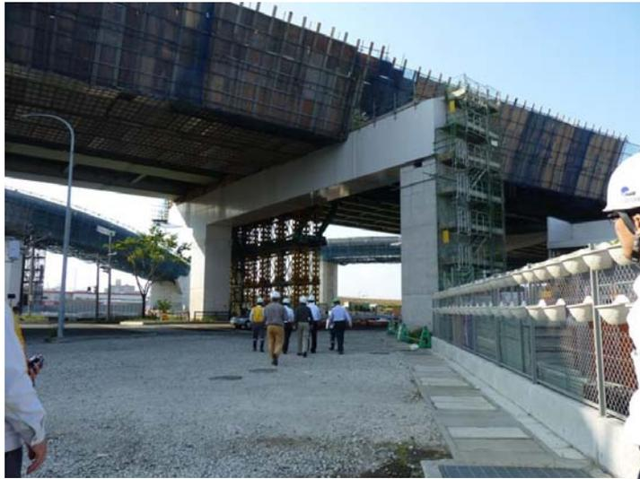
Fig. 2 Two-column frame, Pier 56, Sendai-Tobu Viaduct
