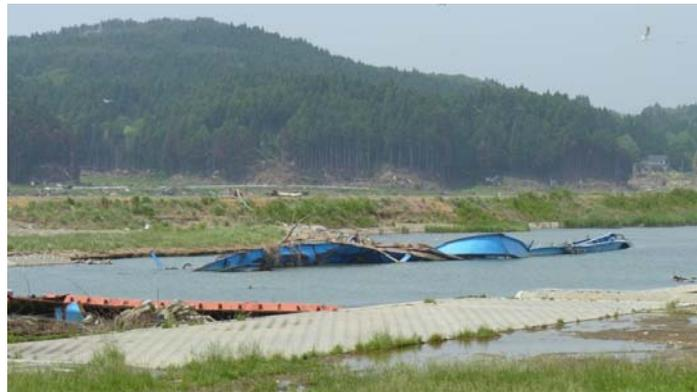
Fig. 7 Girders from Koizumi Bridge 400 m upstream in Tsuya River channel (photo: E. Monzon)
