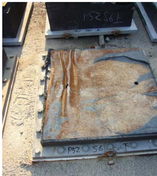
Fig. 4 Damaged elastomeric bearing from Pier 52 Sendai-Tobu Viaduct (photo: I. Buckle)
