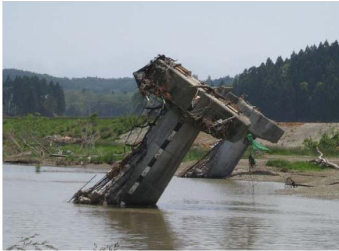
Fig. 8 Damaged piers of the JR Rail Viaduct crossing the Tsuya River (photo: S. Dashti)
