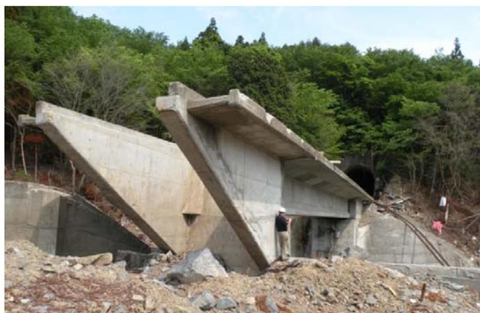
Fig. 10 Exposed wingwalls of JR Rail Bridge 100m upstream from Nijyu-ichihama Bridge due to loss of approach embankment (photo: D. Frost)
