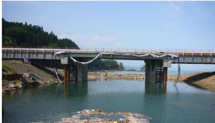
Fig. 9 Loss of backfill on both approaches to single-span Nijyu-ichihama Bridge (photo: I. Buckle)
