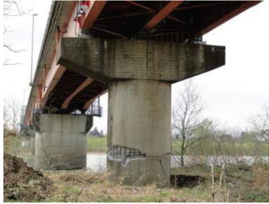
Photo 1 Flexure-shear failure of columns due to termination of longitudinal bars with insufficient development (Fuji Bridge) (courtesy of Dr. Hoshikuma, J., PWRI)
