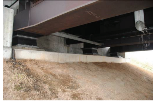
(b) Deck end supported by three elastomeric bearings
