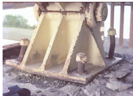
(b) Pull-out of anchor bolts due to rocking response of a lower bearing
