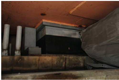
(a) An elastomeric bearing without damage
