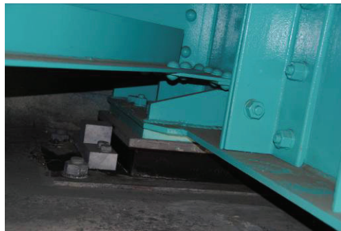
Photo 8 Elastomeric bearings which were set for replacement of original steel bearings suffered no damage, Sendai Bridge
