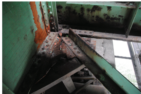
(b) Disconnection at the end of a lower brace
