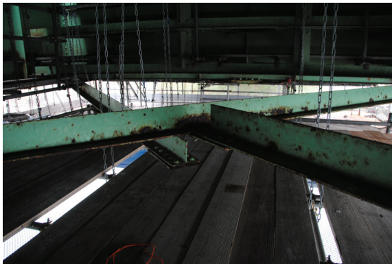
(a) rupture of a lower brace
