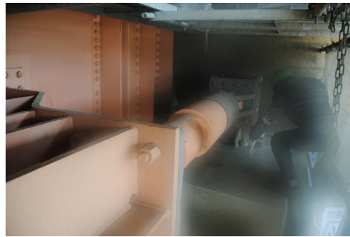
(b) A damper for seismic retrofit
