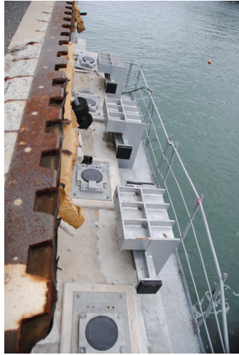
(c) Steel bearings and stoppers on P10
