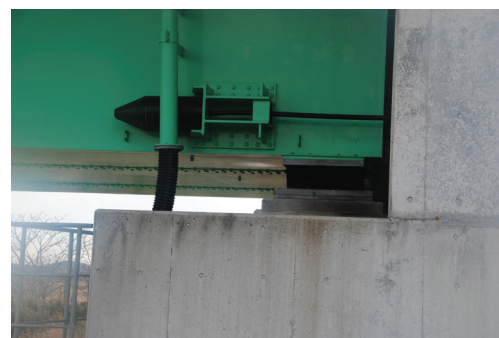
(b) Elastomeric bearing without damage
