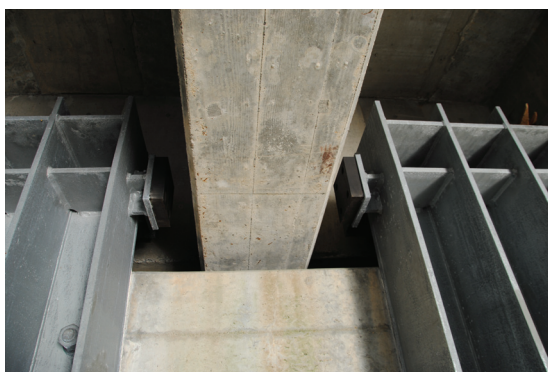
(a) Longitudinal and transverse stopper at A2
