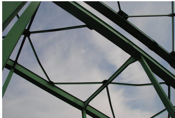
Photo 5 Rupture and buckling of upper braces, Tennoh Bridge, National Road No. 45
