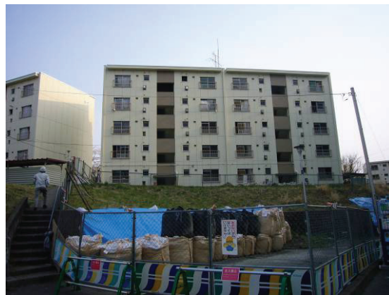
Photo 3 Overview of the apartment inclined and the retaining wall collapsed partially
