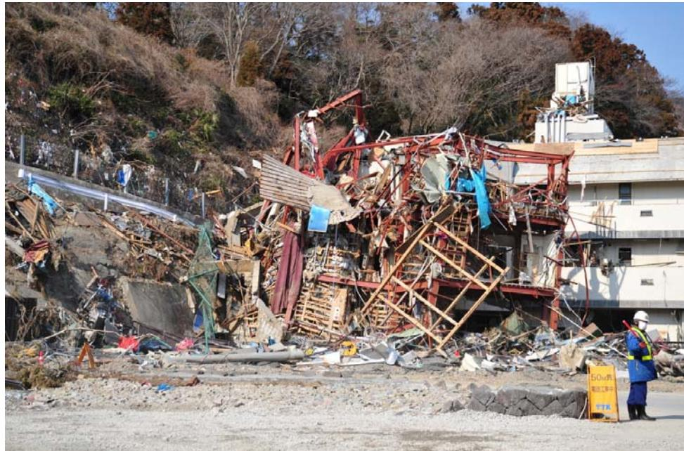
Fig. 1 Total destruction, deformation and movement of steel structures in Onagawa town, Japan 2011
