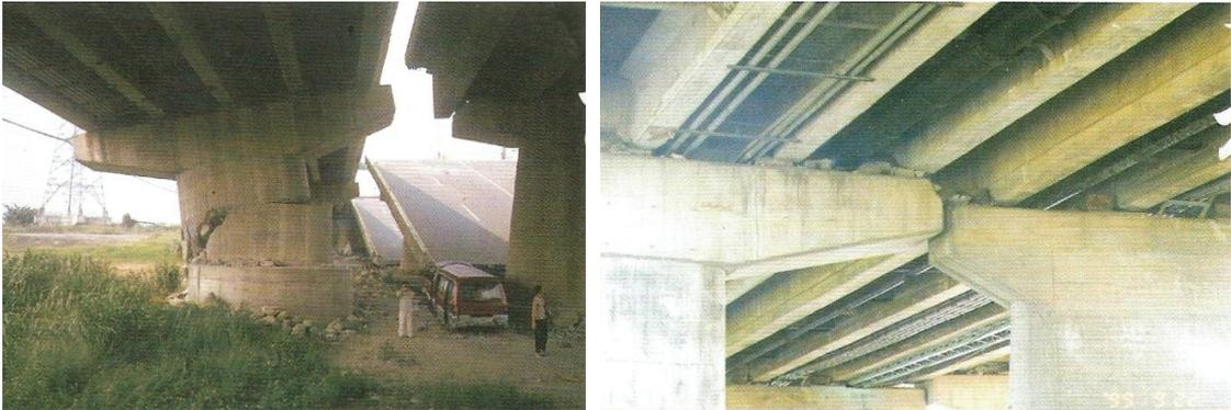
Fig. 1 (Left) Collapsed spans and damaged piers of the Wu-Shi bridge at the third span
