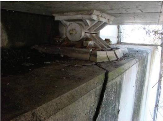
Photo 3 Damage of Pier Top
