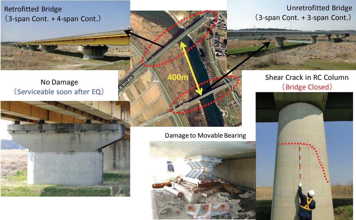
Photo 6 Comparison of Seismic Performance between Adjacent Two Bridges (Nakagawa Bridge and Kunita Ohashi Bridge)
