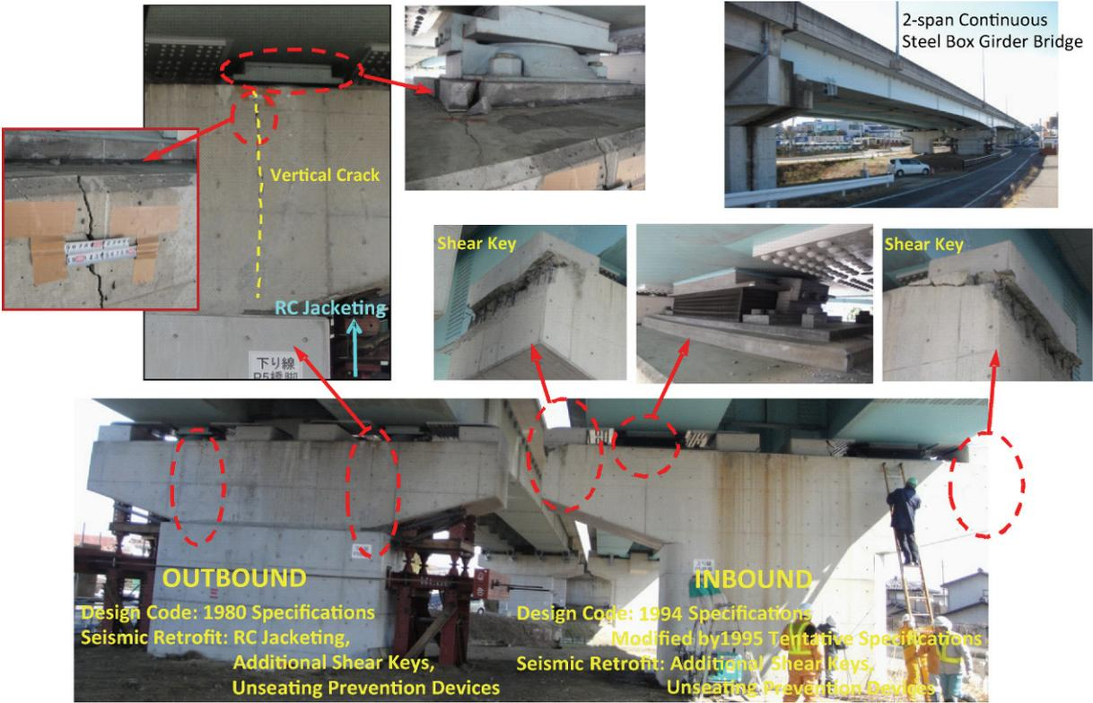
Photo 7 Comparison of Damage Mode between Adjacent Two Bridge Columns (Kameda Ohashi Bridge)
