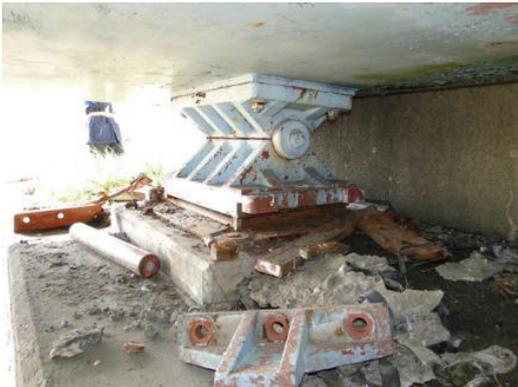
Photo 2 Damage of Steel Bearing Support
