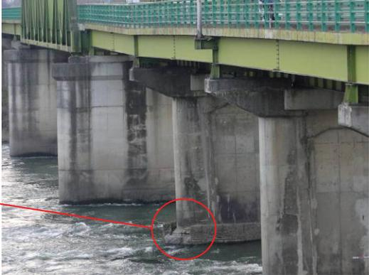
Photo 4 Residual Inclination of Substructure and Damage of Pile Cap for Caisson Foundation
