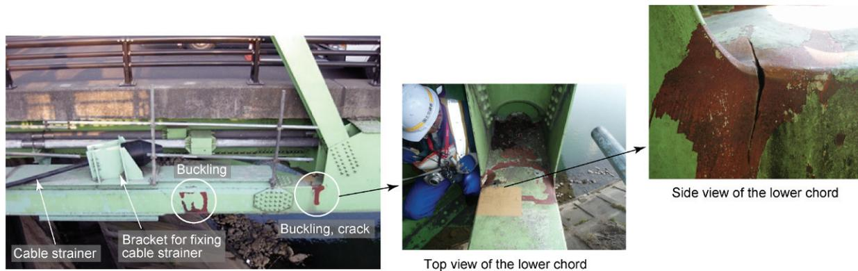
Photo 8 Damage of the lower chord of truss bridge (Osaragi Ohashi Bridge)
