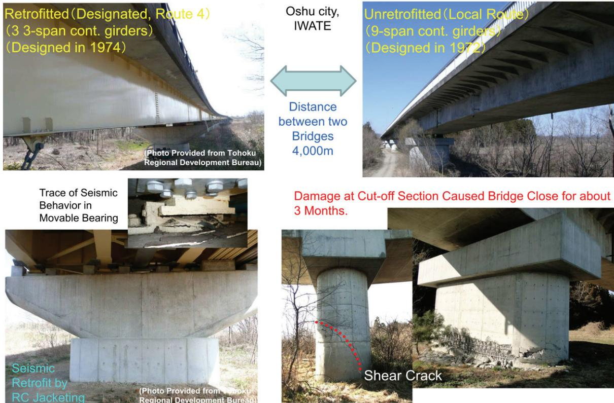
Photo 5 Comparison of Seismic Performance between Adjacent Two Bridges
