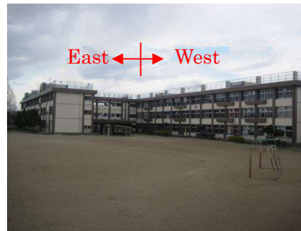
Fig. 2 North view of H school building
