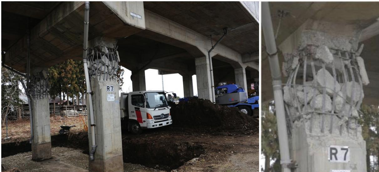
Photo. 1 The damaged columns of an elevated bridge of the Tohoku Shinkansen (Takahashi and Goto 2011)
