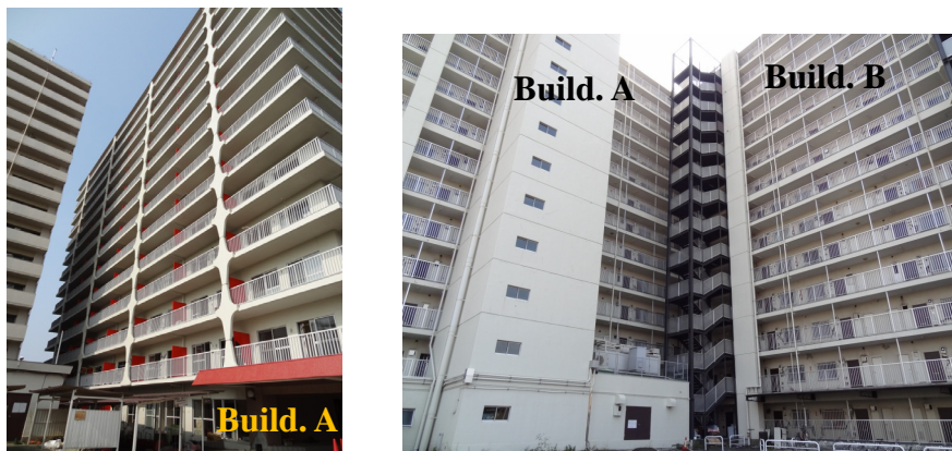
Photo 1 Exterior appearance of the damaged housing complex
