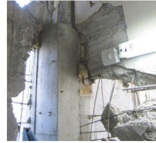
Photo 17 Later reinforced column of the penthouse
