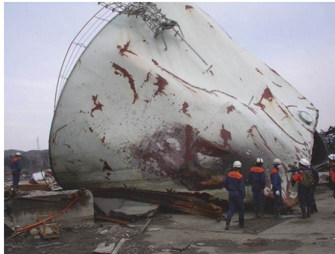
Photo 2 Oil storage tank drifted and collapsed by the Tsunami
