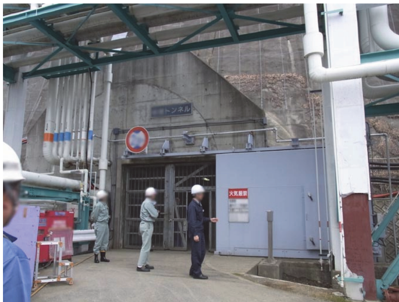
Photo 13 Door of the underground rock cavern oil tanks
