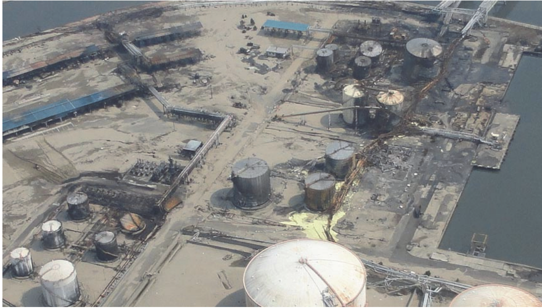
Photo 4 Burned-out section in a refinery
