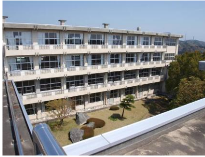
Fig. 2 Overview of Building “A”
