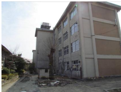
Fig. 4 West side view of Building “A”
