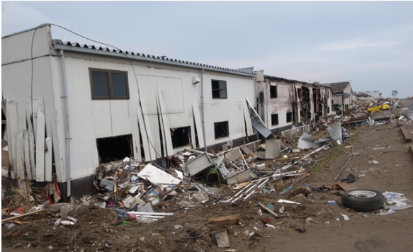
(b) Broken facilities on the river bank side (in the south area)
