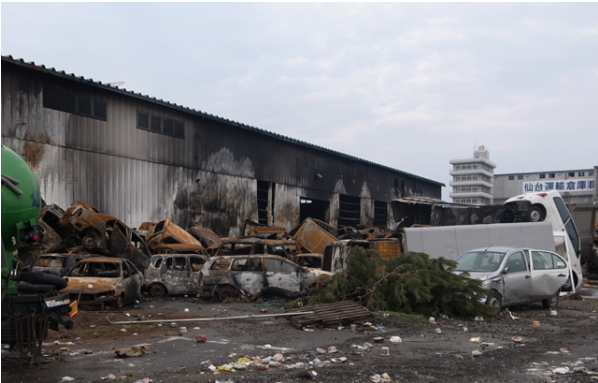
(b) Piles of rubble such as vehicles were swept away toward the building, causing a fire
