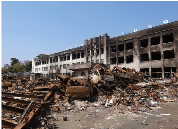
(a) Burnt-out site on the south side of Kadonowaki Elementary School
