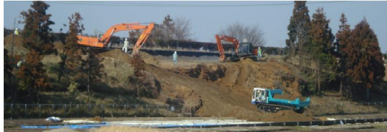
(b) Toe sliding failure under urgent repairing work on March 13
