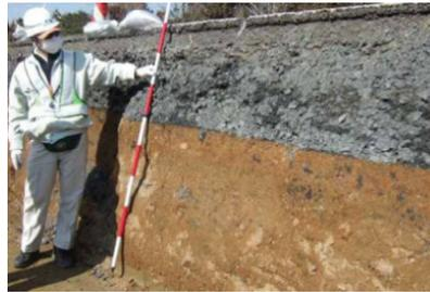
Photo 2 View of pavement and gravelly fine sand layer
