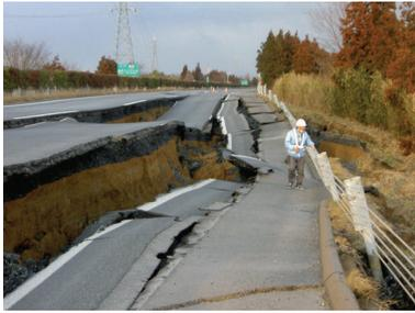
(a) Sliding failure around crest
