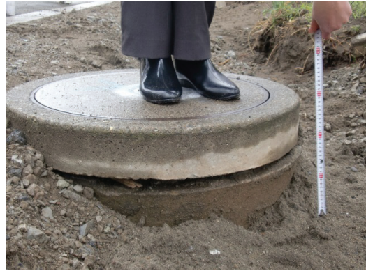
Figure 23 Uplifted manhole
