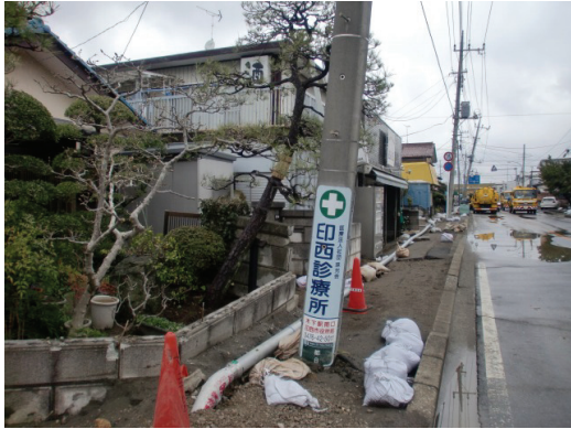
Figure 22 Inclination of power poles
