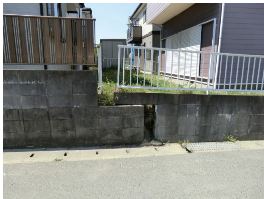
Figure 14 Subsidence damage
