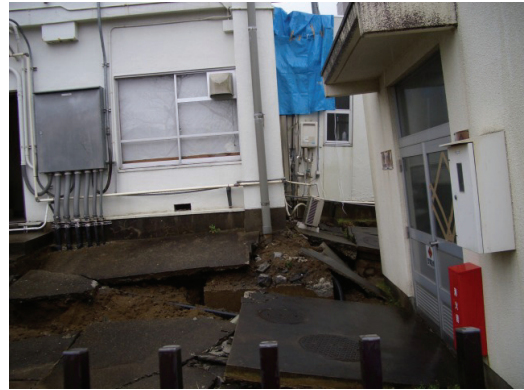
Figure 5 Attached building separated from the main building
