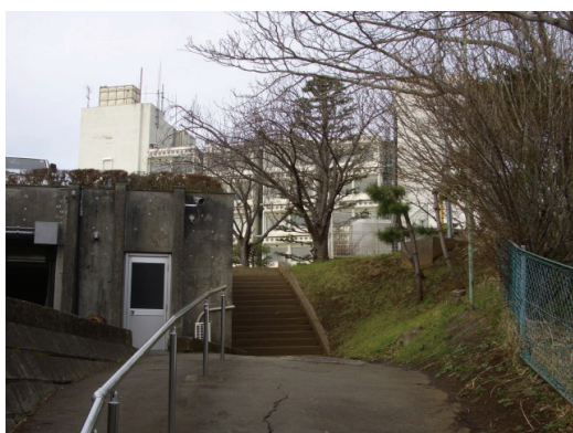
Figure 30 K-NET station and Sakura city hall on the hill.
