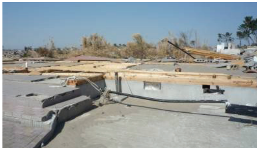
Fig. 25 Movement and complete washed away (left: wood house, right: steel building)
