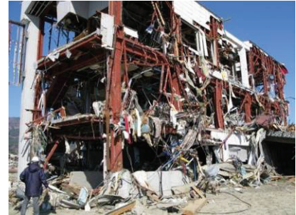
Fig. 28 Story collapse of 1 st story (left), out-of-plane wall deformation (middle) and washed out of claddings (right)
