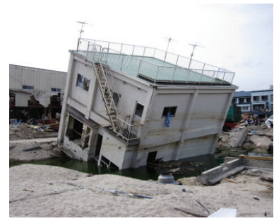
Fig. 27 Tilting by scouring
