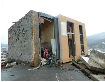
Fig. 26 Overturning (left: reinforced concrete building, right: steel building)
