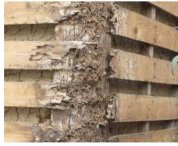
Fig. 7 Fallen down of finishing (bio-deterioration)
