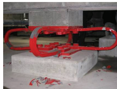
Fig. 20 Yielded steel damper
