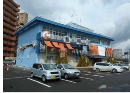
Fig. 15 Collapse of mid-story
