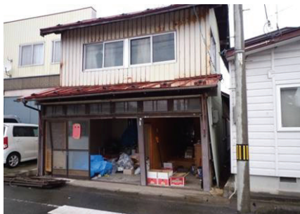
Fig. 5 Inclination of 1 st story
