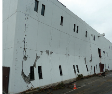
Fig. 28 Story collapse of 1 st story (left), out-of-plane wall deformation (middle) and washed out of claddings (right)
