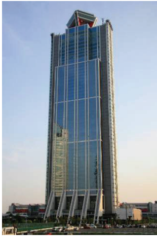
Photo 2 55-story steel office building (Osaka Bay)
