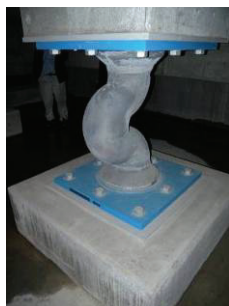
Fig. 21 Lead damper cracked
