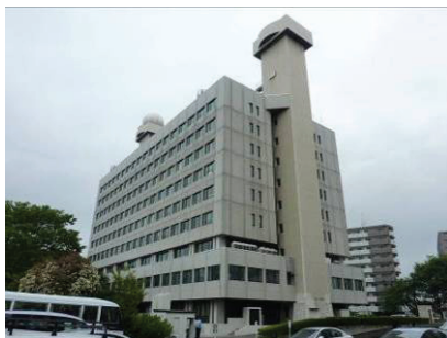
Fig. 19 Seismically isolated building performed well
