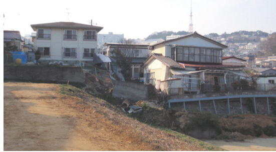
Fig. 24 Ground transformation by sliding
