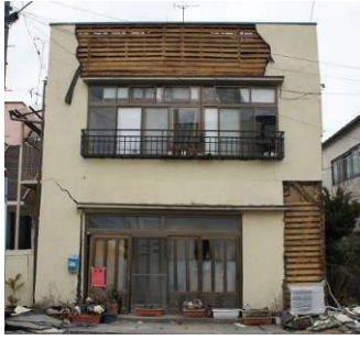
Fig. 7 Fallen down of finishing (bio-deterioration)
