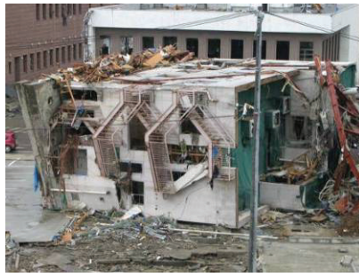
Fig. 26 Overturning (left: reinforced concrete building, right: steel building)
