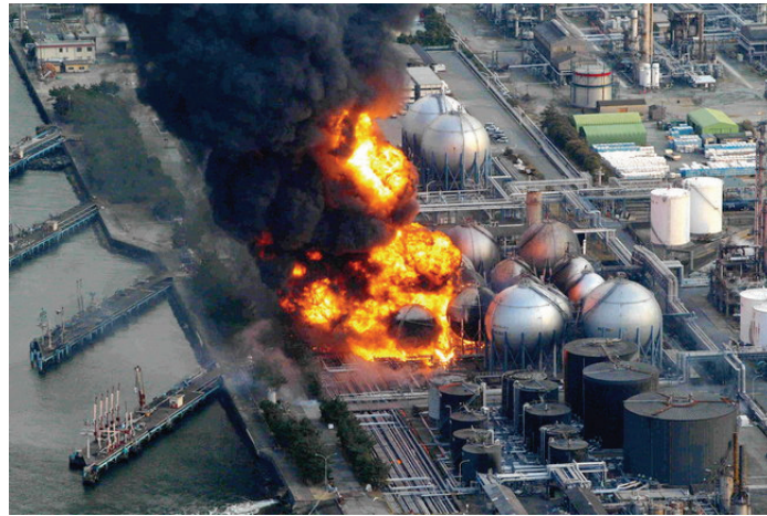
Photo 1 An explosion in flames of a liquefied petroleum gas tank (Asahi.com 2011)
