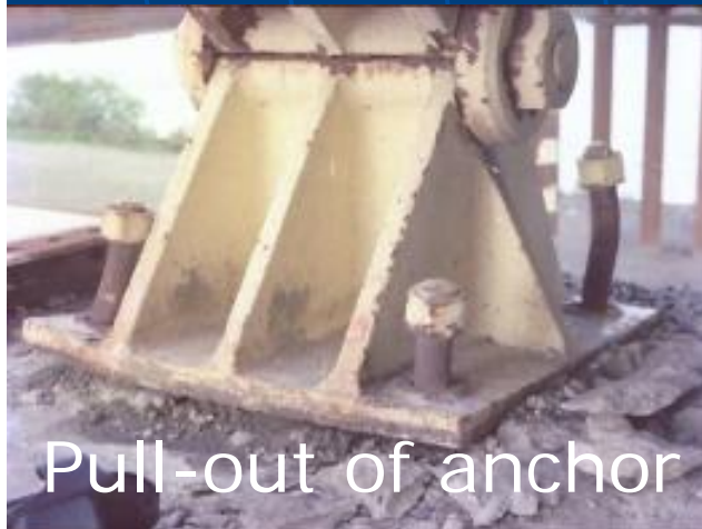
Damaged side stoppers
