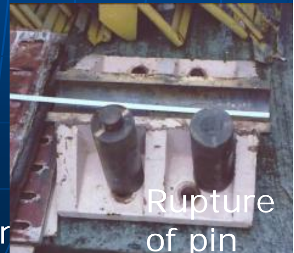
Failure of pier at bearing
