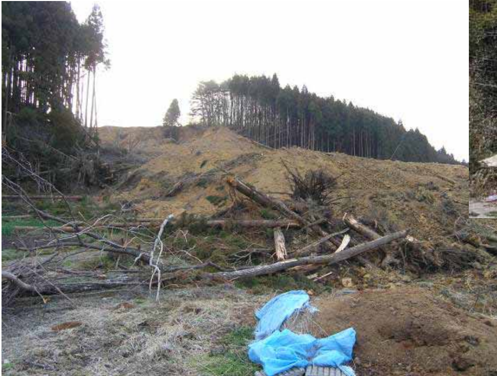
Failure of natural slope at Hanokodaira Shirakawa City, Fukushima Prefecture
