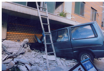
Figure 1. Story failure of a soft-first-story building
