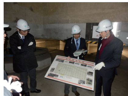
Photo 2. Observation of the seismic isolation retrofit of the Central Gov't Bldg. No.3 (MLIT).
