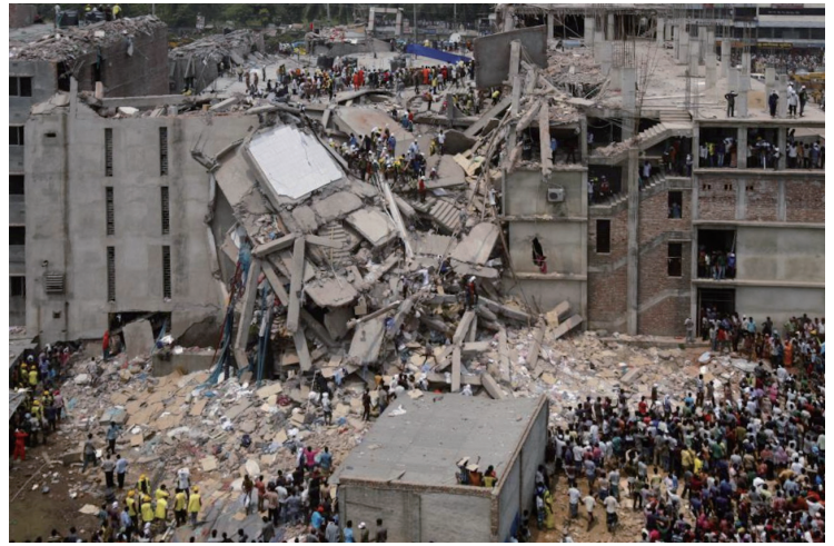
Rana Plaza Collapse in 2013
