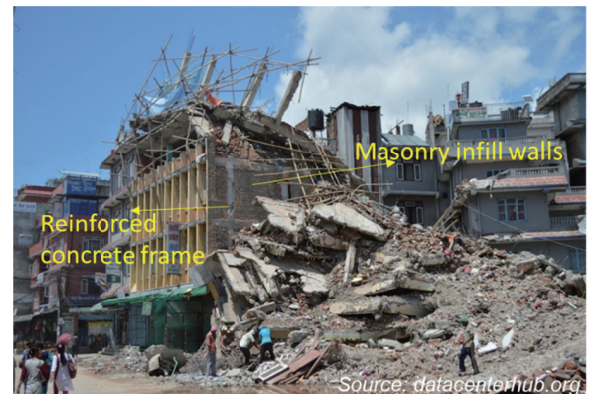
Fig.1 Damage to reinforced concrete buildings with masonry infill in Nepal EQ 2015. Source of photo [1]
