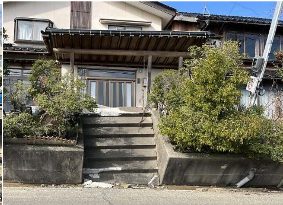
図63 内灘町西荒屋ハ6-41 (36.678928, 136.668547E, 方位角314.9479°)
