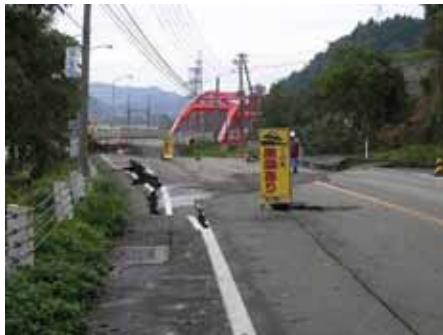
Fig. 3.1 Differential settlement between road embankment and bridge
