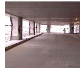
Fig.7 Inner Space under Construction
