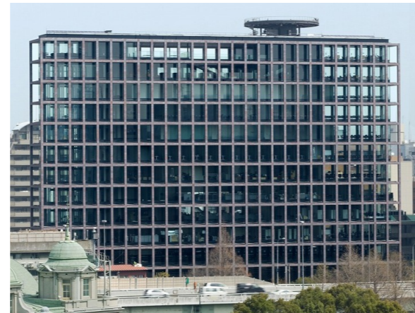
Fig. 1: Appearance of building
