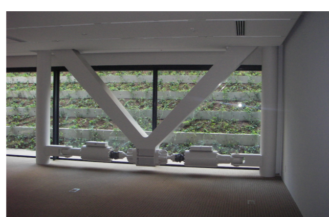
Fig. 6: Oil dampers intensively provided on vibration control story
