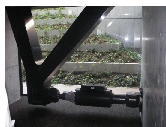
Fig. 6: Oil dampers intensively provided on vibration control story
