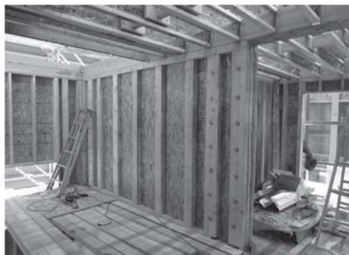
写真3 Mid-ply shear wall
