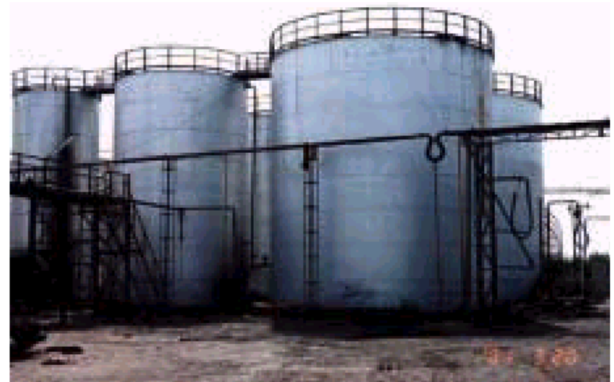
(b) Non-damaged oil tanks at Trisuns Plant
