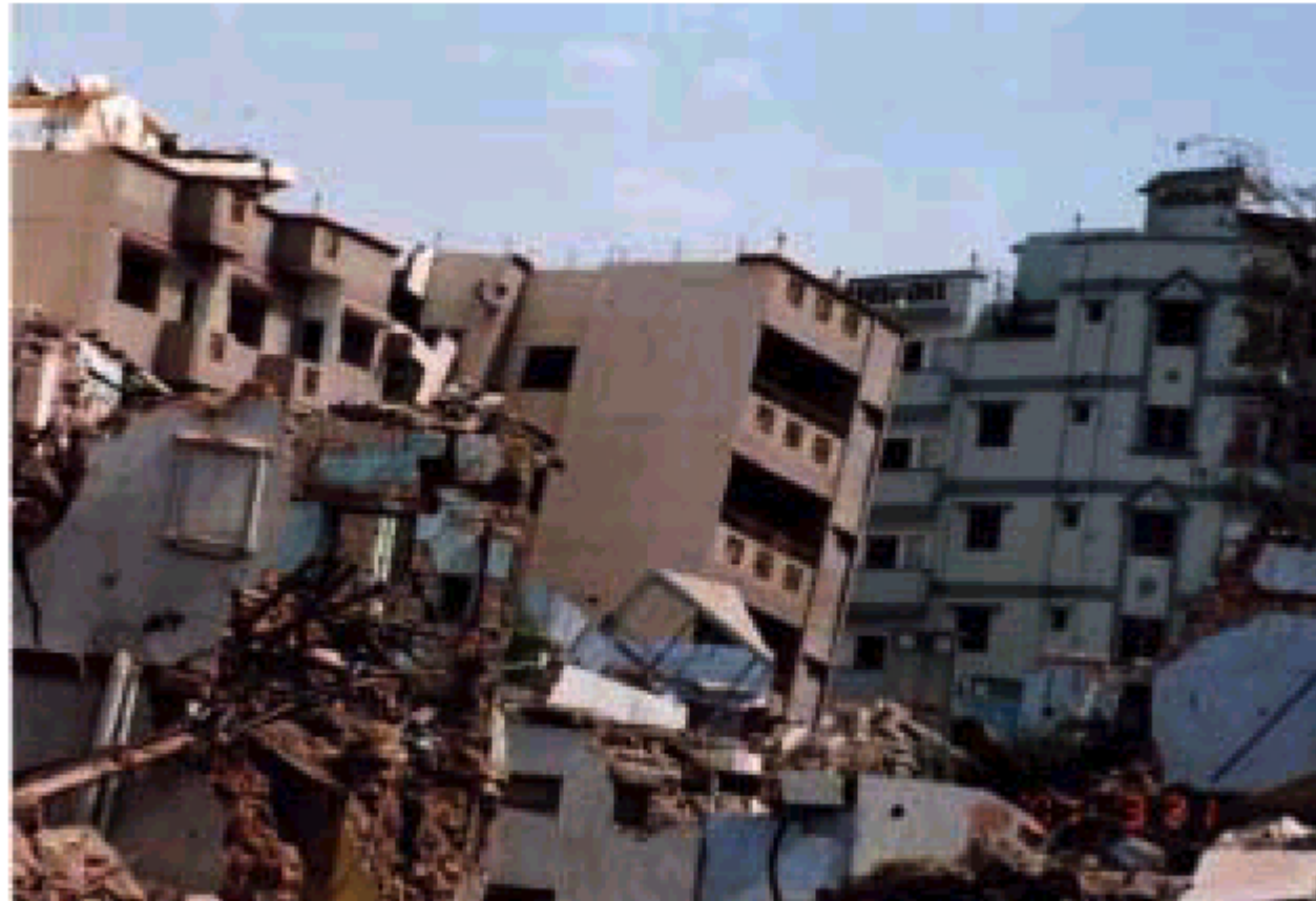
Figure 30 Collapsed Apartment blocks are ground floor in Bhuj
