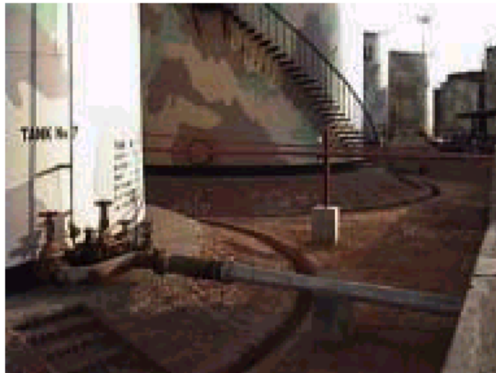
(a) Damaged Tanks at Oil India
