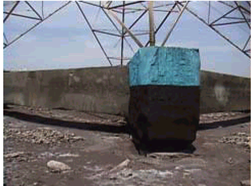
Figure 19 Damaged pylons near Hadakia Bridge
