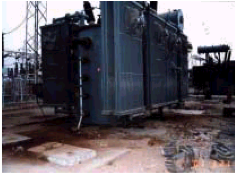
Figure 20 Displaced transformers and damaged breakers at Anjar sub-station
