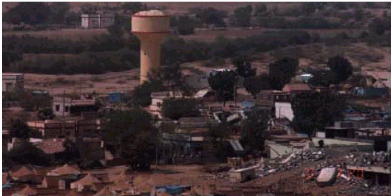
Figure 29 Non-damaged typical elevated water tank in Bachau
