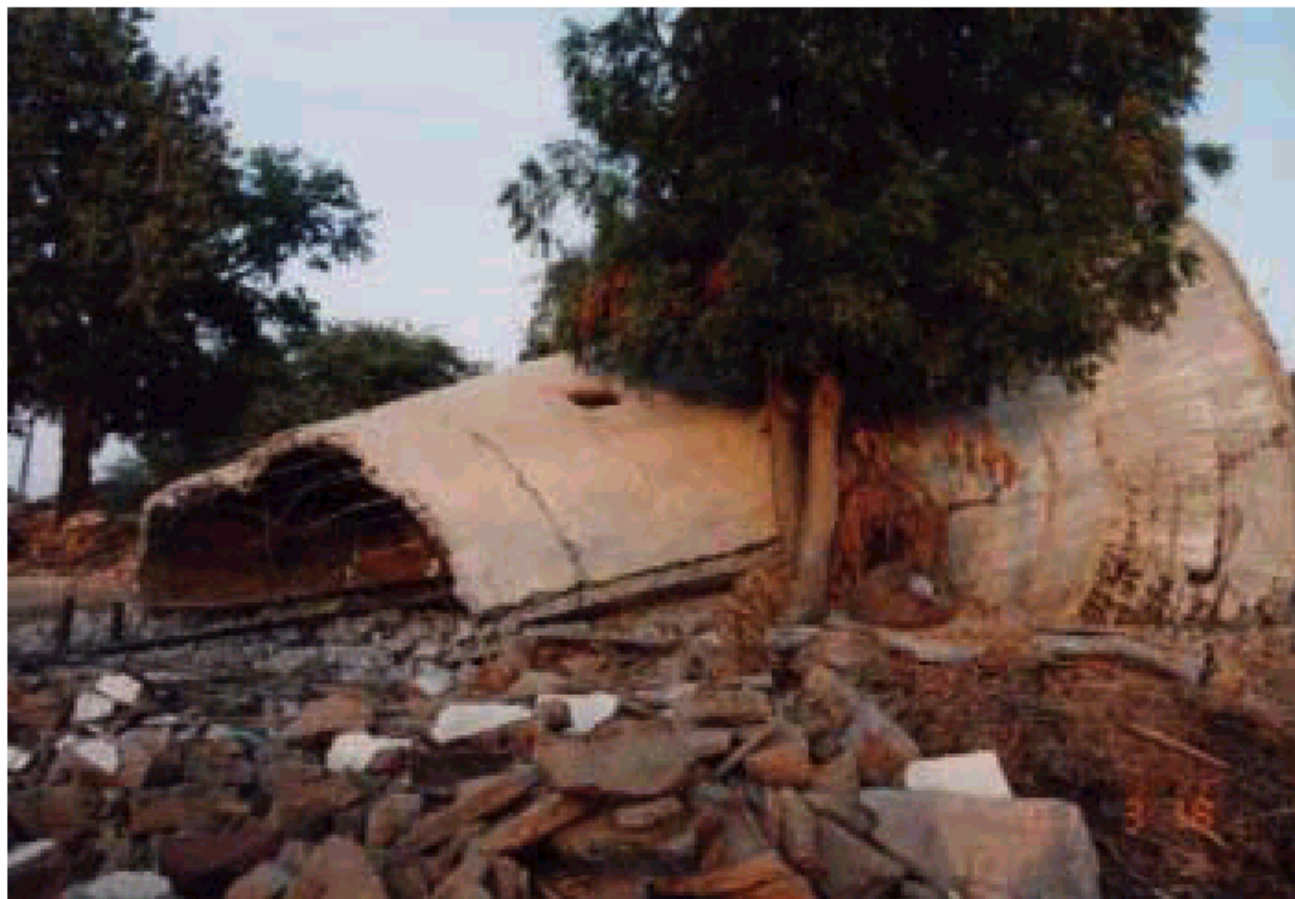
Figure 30 Collapsed water tank in Chobari village
