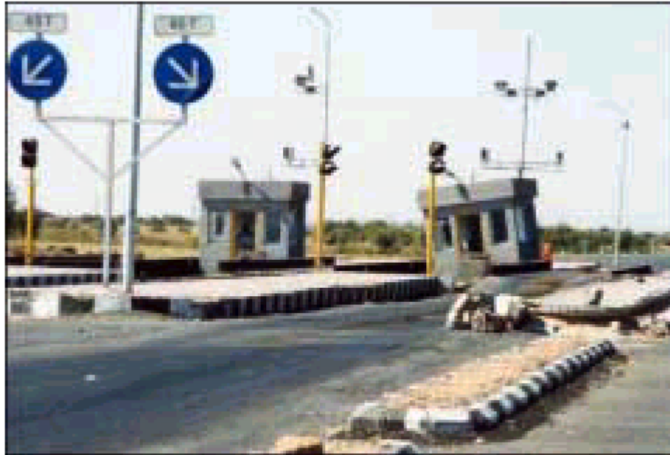
Figure 17 Damage to toll gates and settlement of bridge embankments
