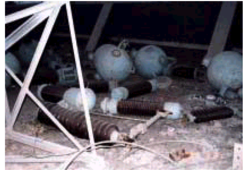
Figure 20 Displaced transformers and damaged breakers at Anjar sub-station
