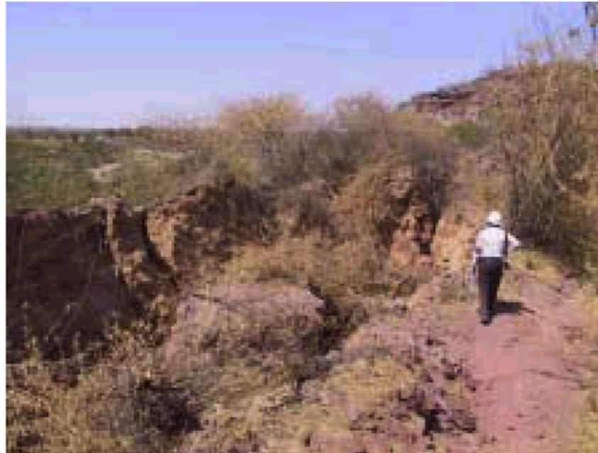
(a) Chang Dam
