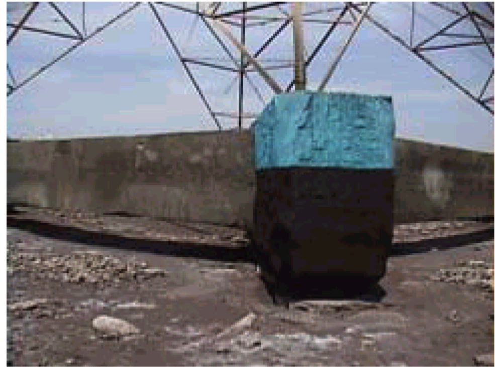
Figure 19 Damaged pylons near Hadakia Bridge
