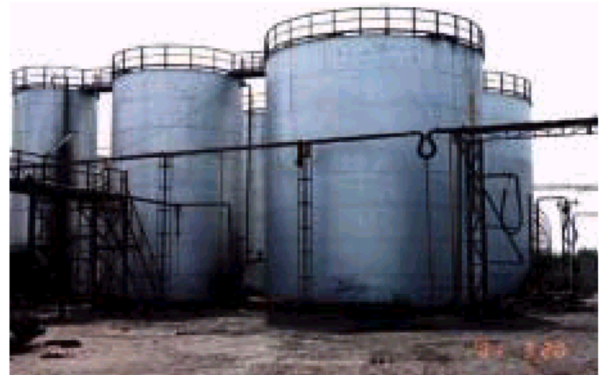
(b) Non-damaged oil tanks at Trisuns Plant
