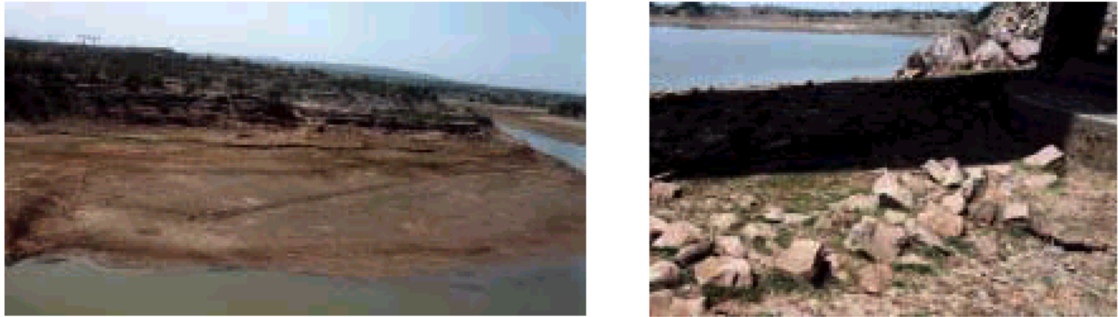
Figure 26 Settlement and lateral spreading in the vicinity of Rudramata Bridge
