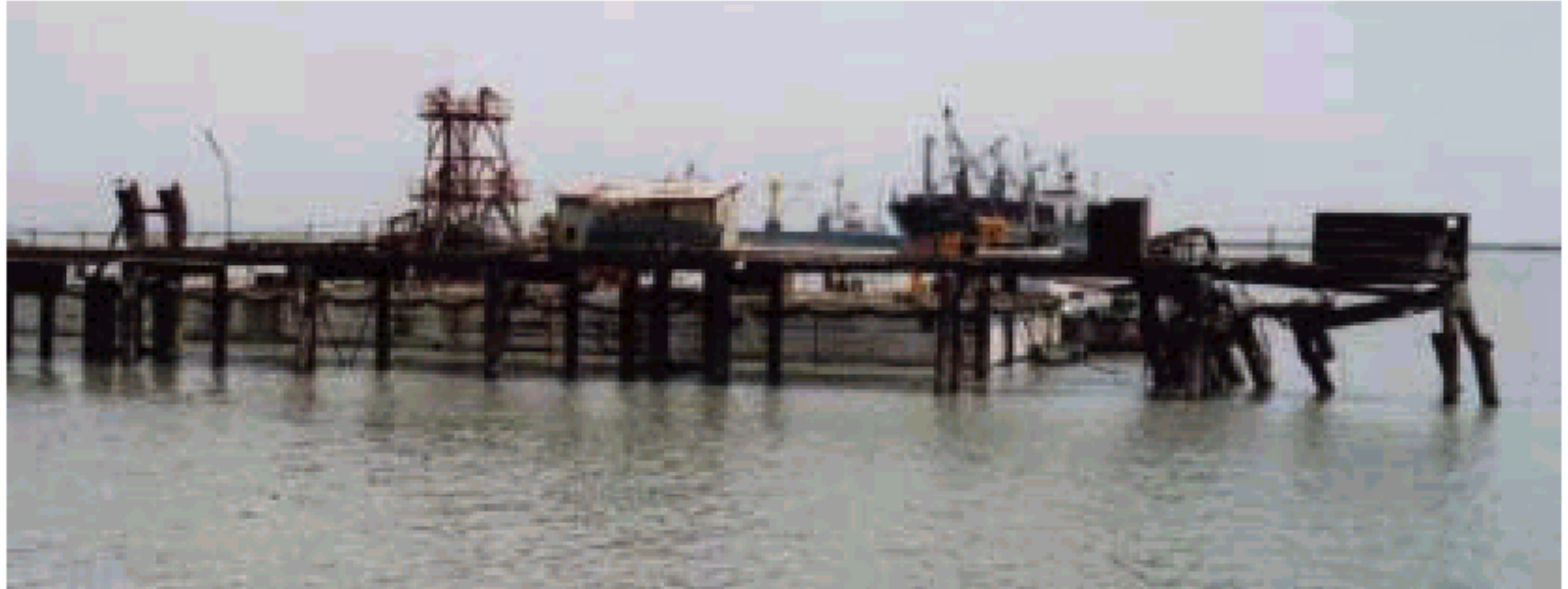
Figure 15 A view of damaged oil jetty at the Kandla port on March 19, 2001.
