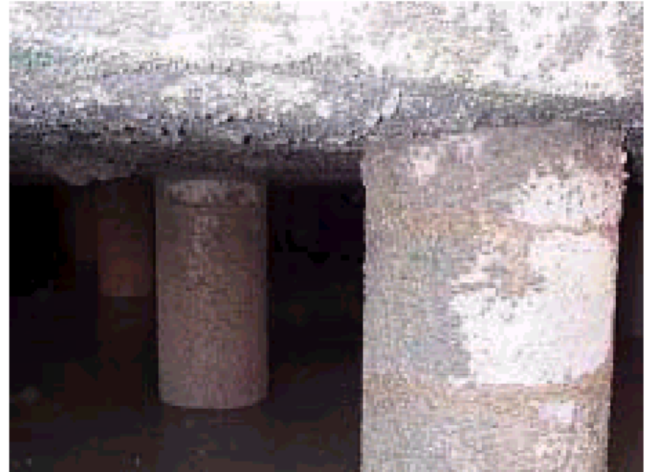
Figure 14 Cracking of piles at Kandla port
