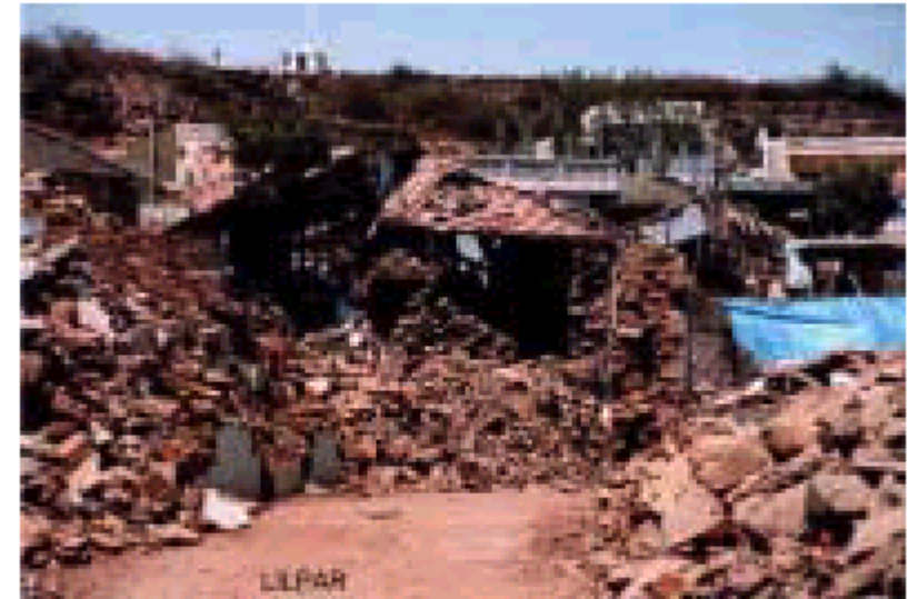
Figure 28 Examples of damage to masonry buildings in Bachau and Lilpar
