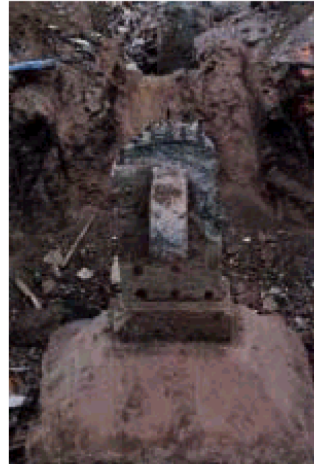
Figure 29 Partially collapsed Mansi Apartment Complex in Ahmedabad and its footing
