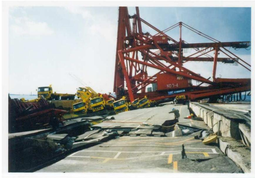
Photo 1 Damage to a quay wall at the Port of Kobe during the 1995 Hyogo-ken Nanbu Earthquake
