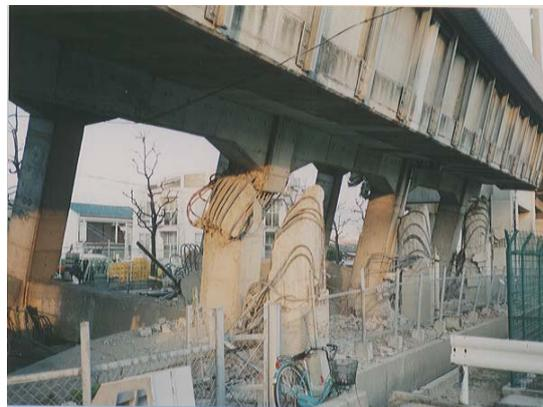
Photo 1 Damage of RC rigid frame structure
