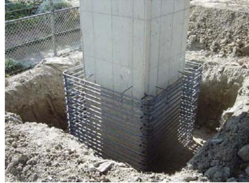
Photo 2 Arrangements of retrofitting reinforcements
