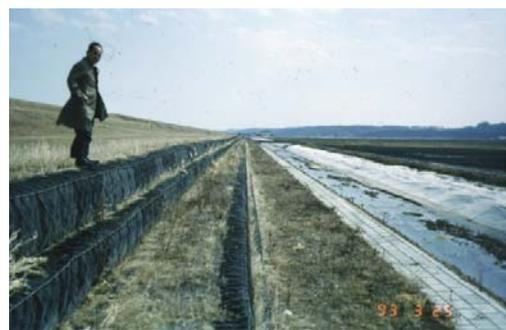
**Fig. 33 Gabion at the toe of the Tokachi River dike**
