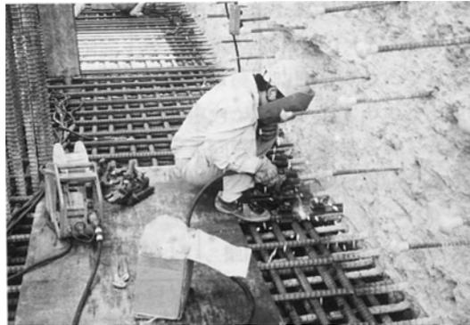
Fig.8 View of enclosed welding
