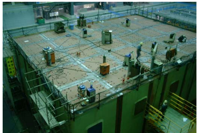
Fig.4 Shaking table (welding of 32 blocks
